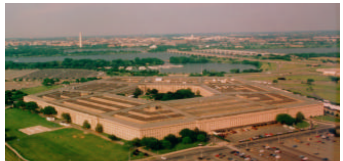
Pentagon Renovation after 9/11
