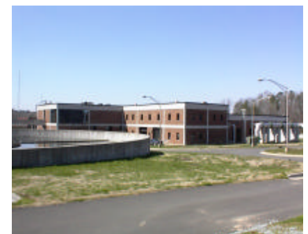
Durham Wastewater Plant
